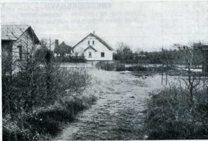
Rimmen smalspor station
